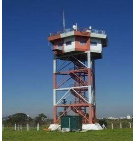
Fig.01. ACA tower room at 25 m high above ground level (author)
